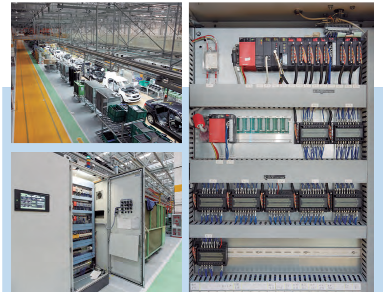
Inside the 2nd factory of FAW Car Co., Ltd., and installed CC-Link devices.
